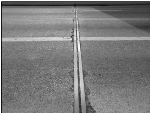
COMPRESSION JOINT AT BENT LC4 (Typ. of compression joints)
