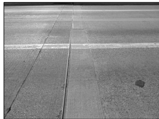
POURABLE JOINT AT NORTH ABUTMENT
