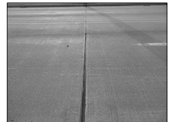
STRIP SEAL JOINT AT BENT LC7
