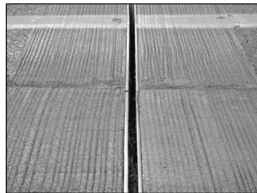
COMPRESSION JOINT AT BENT JC4 (Typ. of compression joints)
